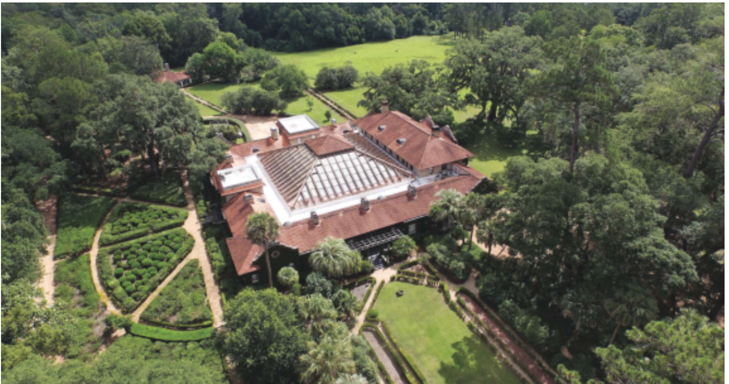
Unlike many plantation homes built in and around Thomasville, Georgia, which were completed in the Classic Revival Style, Millpond Plantation has a Spanish Revival flair. The 38,000-square-foot home consists of 11 fully appointed bedrooms and 10.5 baths. The 3,267-acre plantation is listed with Ben McCollum of The Wright Group.
